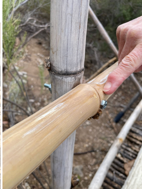
Bamboo can be thick enough to drill holes in and use nuts and bolts to secure it to a post
